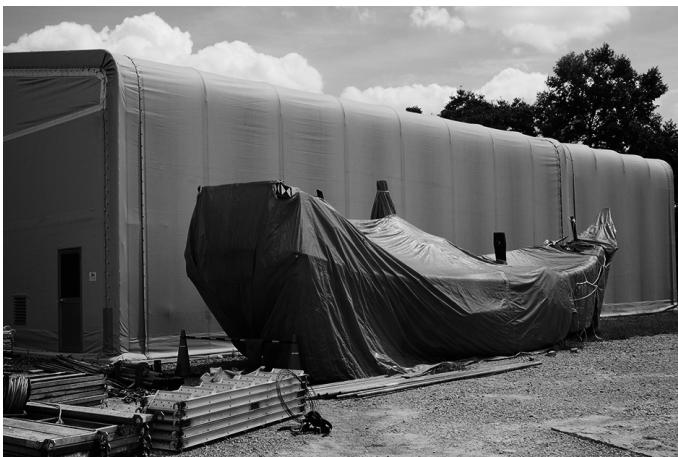
The new 'temporary' shed, with a small ship waiting to be moved (Matthews, 2014)
